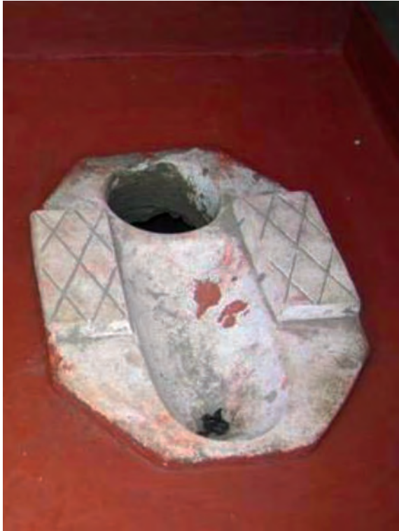
An EcoSan toilet pan – The urine is diverted into a plastic storage tank.
