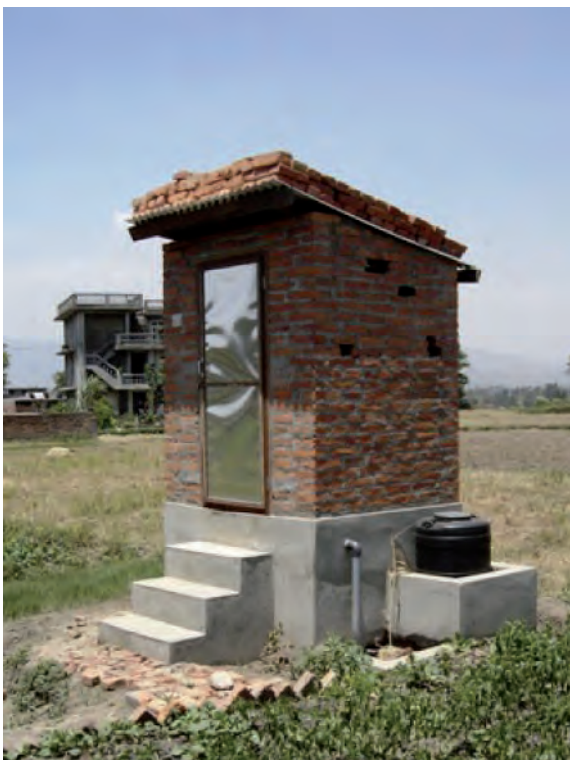
An EcoSan toilet in Siddhipur – The dehydration vaults are made of concrete, the superstructure of brick masonry. The urine is diverted into a 100 L PP tank adjacent to the construction
